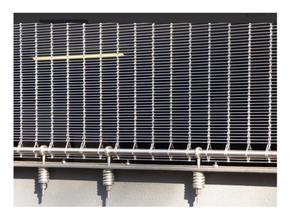
Analog to the top fastening, a round tube is inserted into the cable-rod mesh. The elements are tension with of eye-bolts, for example, on a continuous substructure. The eye-bolts ensure an exact amount of tension. Together with the pressure springs, the mesh is installed with the exact pretension load.
