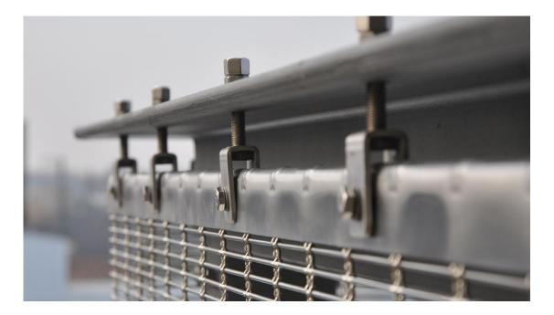
A flat tension profile is provided with clevis screws, which are used to hang the element in the substructure. At the same time, tension is applied to the upper fastening point.
