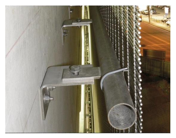
The intermediate mounting is done by the use of wire connector. These run around a tube installed behind the cable mesh and keep it in position when connected to groups of cables from behind. This type of mounting is not visible in the front view.
