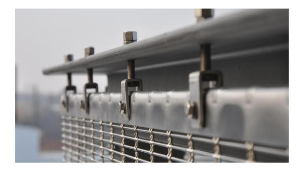
A flat tension profile is provided with clevis screws, which are used to hang the element in the substructure. At the same time, tension is applied to the upper fastening point.
