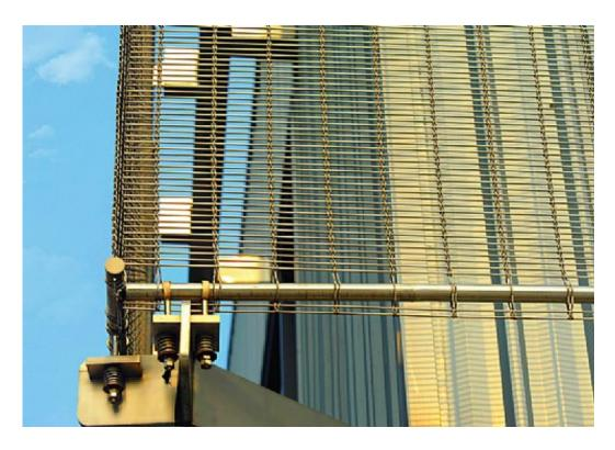
This mesh system is ideal for the dense. And the heavy mesh consists of metal tube, eye-bolt and screws. When preparing the accessories, the metal tube will go through the eye-bolt and the mesh. When installing the mesh, the mesh panel will be tensed by the metal tube and eye-bolts.
