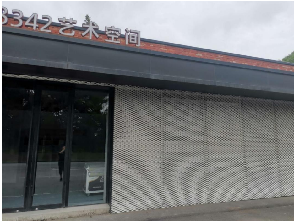
Building facade in Shanghai(1500*3000mm Expanded Metal Mesh)
