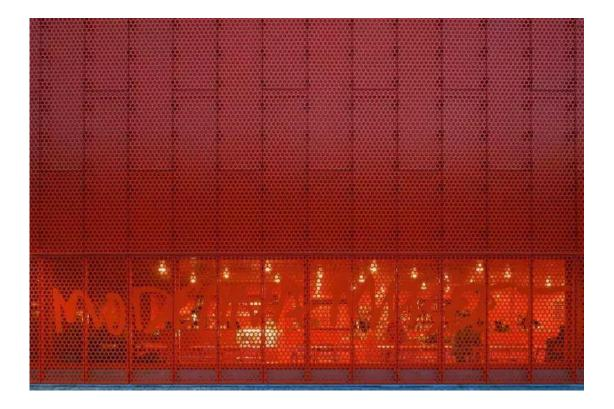
1. Install the perforated metal by bolts, the holes will be drilled during the production of perforated metal or stainless steel perforated metal, then fix the panels on site directly.
